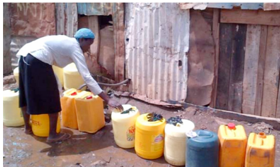
▶ Illegal water connections passing close to an open sewer in an informal settlement in Nairobi
